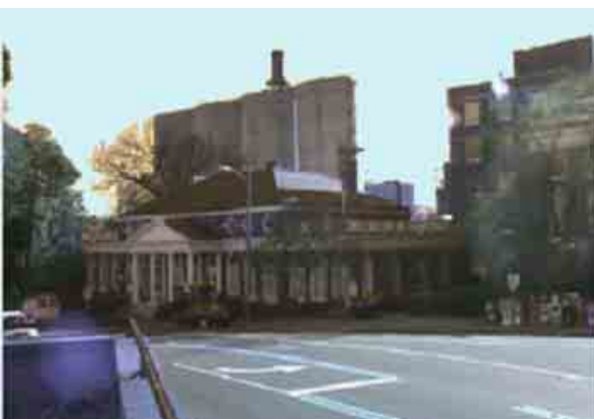
Existing silos as seen from University Avenue.
