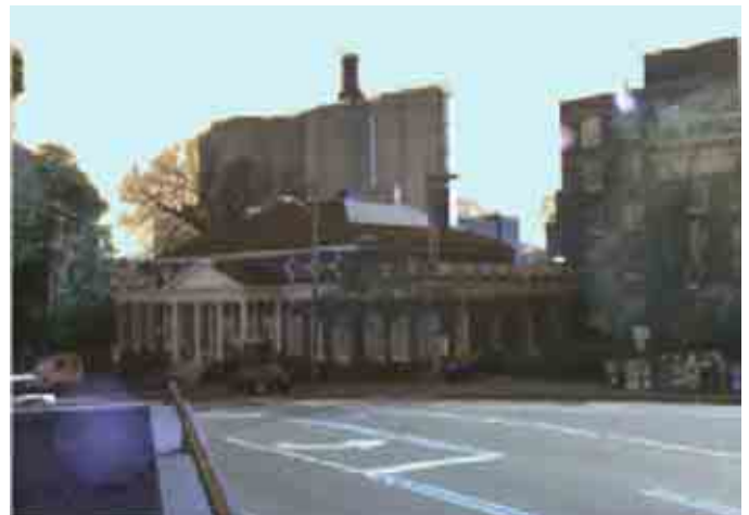
This photo representation shows that the new silo is tucked into space adjacent to the existing silos.
